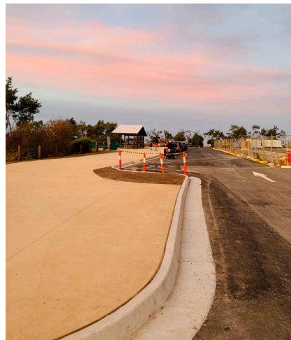
Currumbin Point path and carpark upgrade
