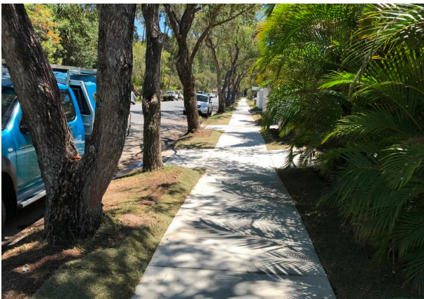
Image: New footpath Carlyle Drive, Currumbin
